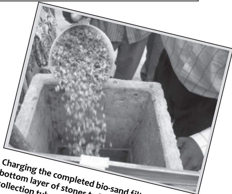
Charging the completed bio-sand filter by pouring the bottom layer of stones to keep the sand out of the collection tube.
