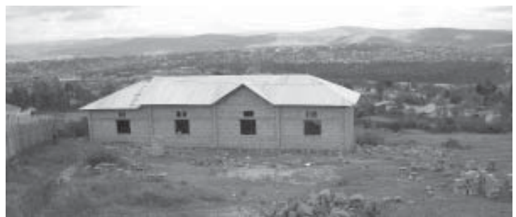
This was built by the July 2007 AGLI workcampers for the street children's program in Rwanda. The blocks were made by the older children who would like to make cement block-making into a business. Because of the considerable amount of firewood used to make bricks, the government has banned the use of bricks.
