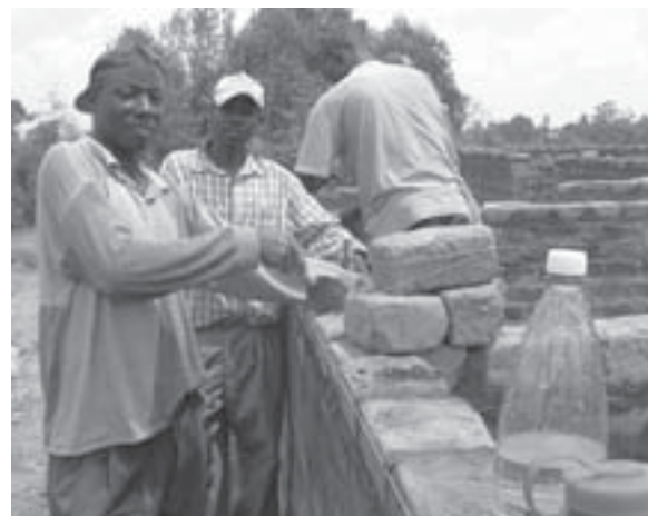
Building the walls at the AVP Peace Center in western Kenya
