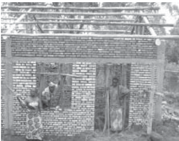
Women working on the new Nyarurambi School
